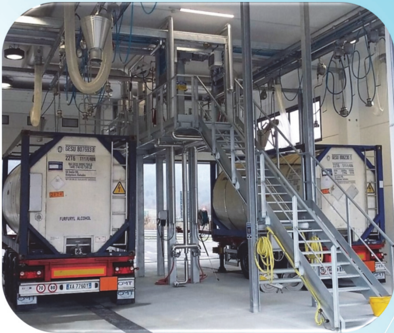
Separate washing lines: for food tanks and chemical tanks.
